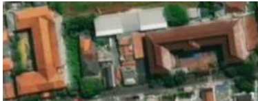
A U-shaped school building
